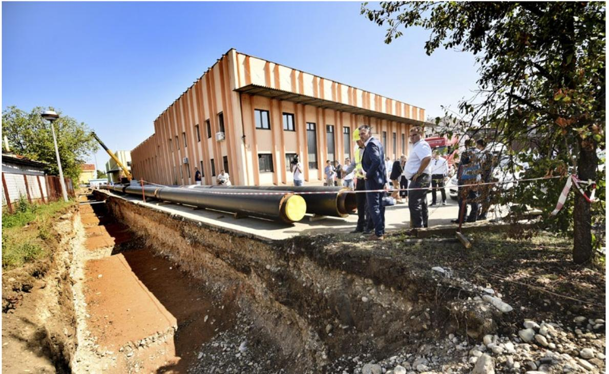
Pipes being laid during the construction phase of the new Banja Luka district energy system.
